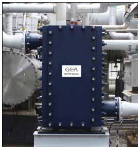
FIGURE 3. The fully welded construction makes the GEABloc heat exchanger well suited for applications that require the high efficiency and compact size of plate heat exchangers, but where conditions exceed the capabilities of gasketed-plate heat exchangers
